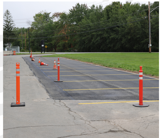
Expanded parking in JSHS front lot
